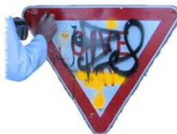
Initial graffiti removal using Graffiti Remover
